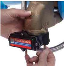
3. Use the wrench to tighten the bolts up to 120 in-lb (10 ft-lb). Do not overtighten.
